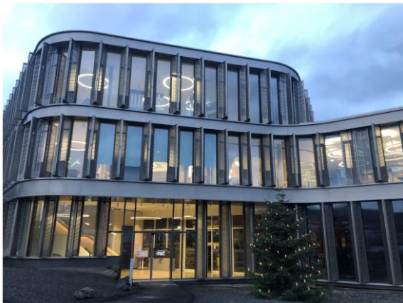
Figure 3: Sustainability also in corporate headquarters WI.com: The facade of the building adapts to the climatic conditions and serves as thermal insulation. Copyright: WIKUS-Sägenfabrik
