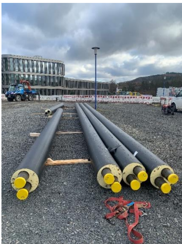
Figure 1: The pipelines are encased in thick insulation to ensure that as little energy as possible is dissipated to the outside. Copyright: WIKUS-Sägenfabrik
