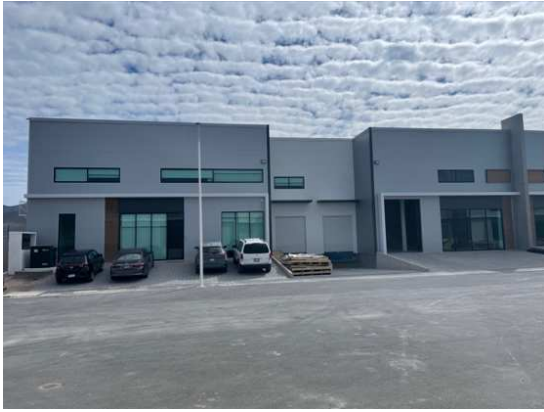
Image 4: A view of the exterior of the newly constructed WIKUS company building in Mexico. Source: WIKUS-Sägenfabrik
